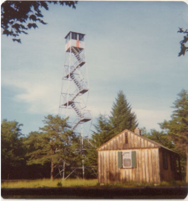
Chapin Hill (R) was erected with funds from Sullivan County. It was also a 60 foot Aeromotor LS40 and stood through the 1970 season. Photo taken in 1974 by Bob Eckler.
